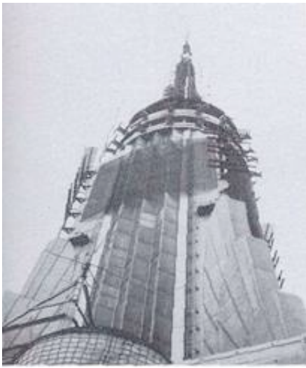
Fig. 4 "Yagi" arrays are for Ch 13
